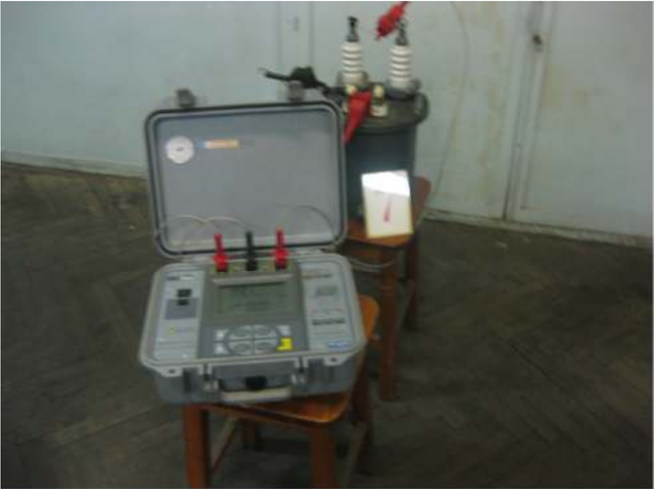
N.7 Determining High voltage transformers insulation systems resistance by meger
