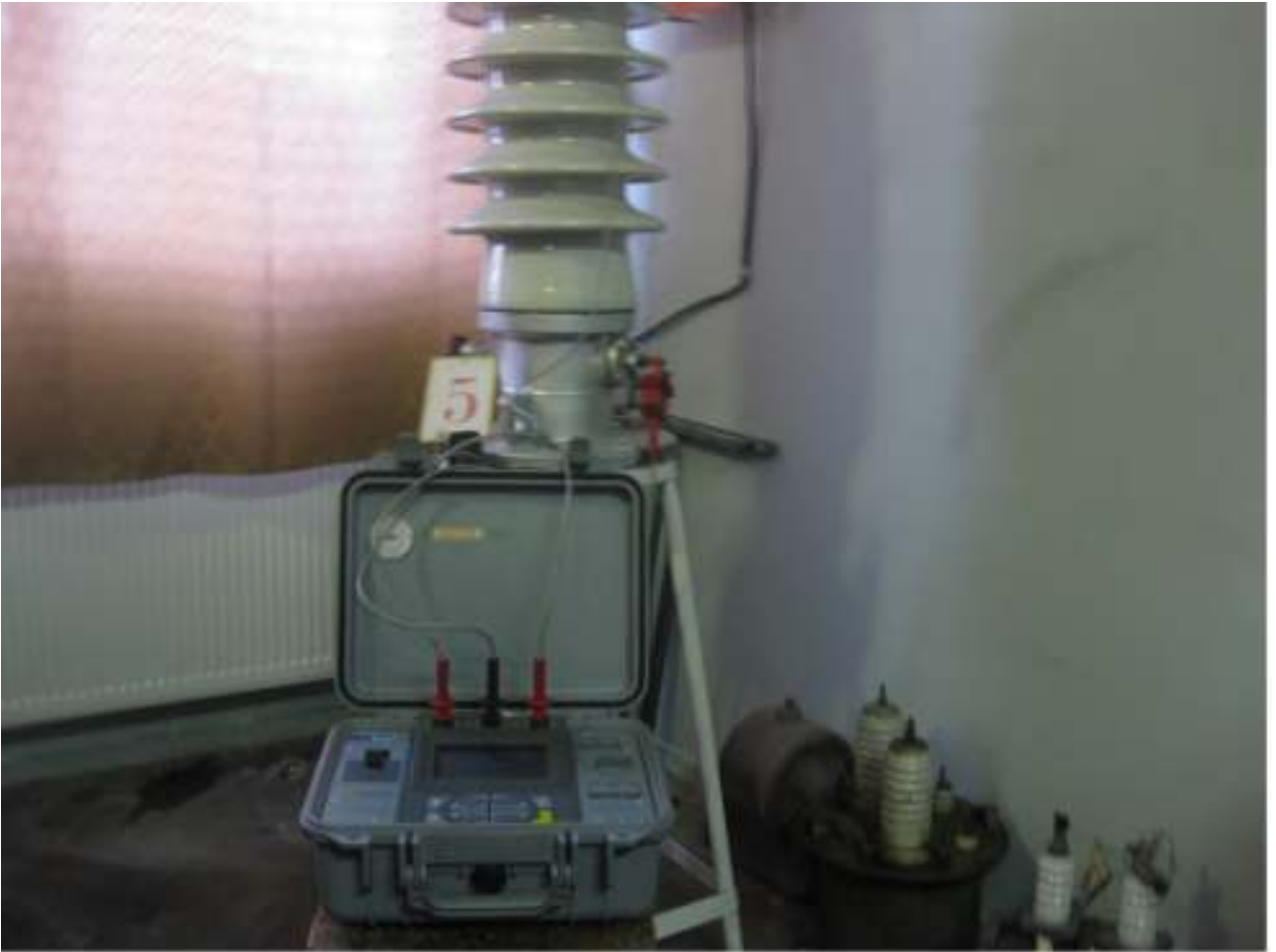
N.5 Determination high voltage bushings insulation systems resistance by meger
