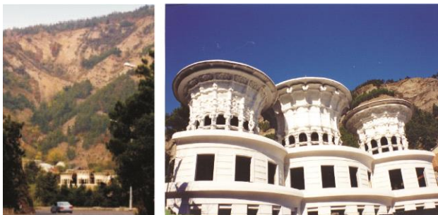
Figure 6: The Palace of Poetry, Tbilisi (1999-2003): (Left) The site context and (Right): Detail of the towers. (Photos: © Shota Bostanashvili Archive, Tbilisi).
