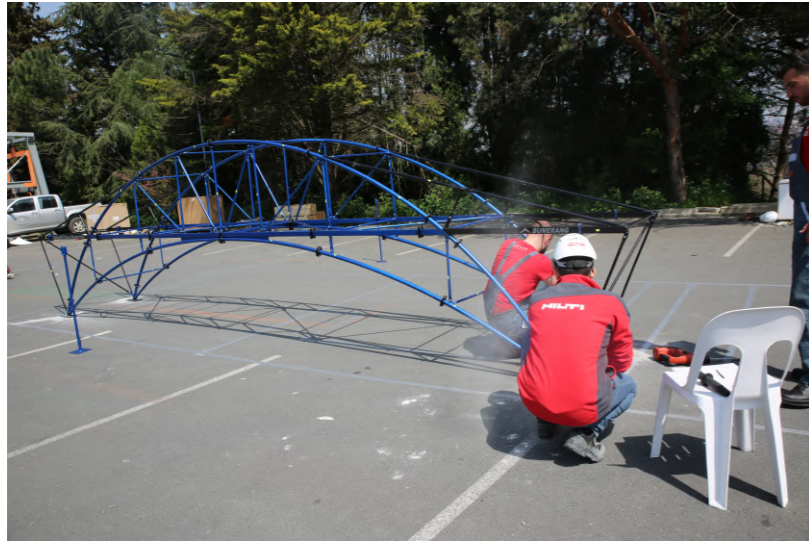
Bridge piers will be fixed
